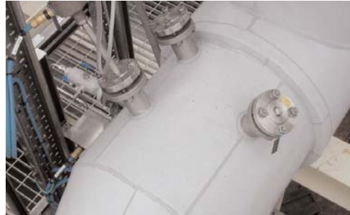
Ulva Shield site-applied to complex spool, including multiple penetrations
