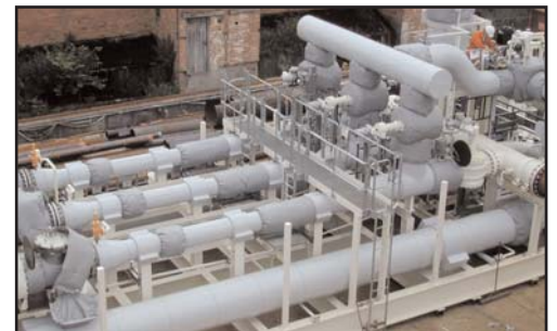
Ulva Shield and Ulva IJS applied to vendor metering skid
