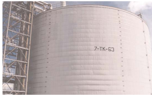
Ulva Shield cladding to propane storage tank 26m high X 55m diameter
