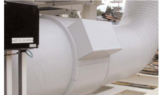
Ulva Shield, (moulded and site applied), to corrosion-protect a hub connector
