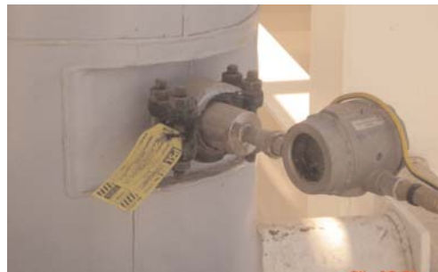
Ulva Shield site-fabricated, recessed penetration detail
